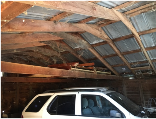
Dillard Ranch - Garage - Roof Decking
