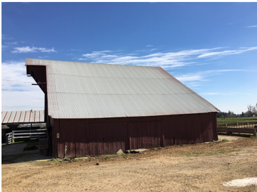
Dillard Ranch - Barn2 - Roof
