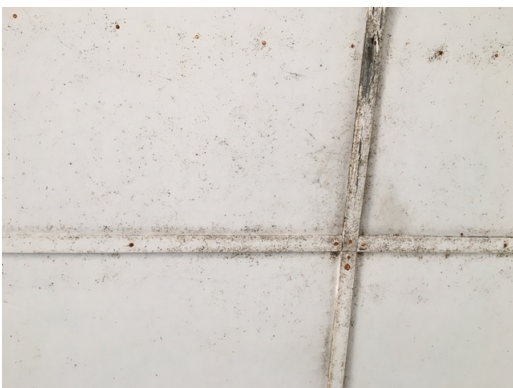
Dillard Ranch - Outbuilding Shed - Ceiling
