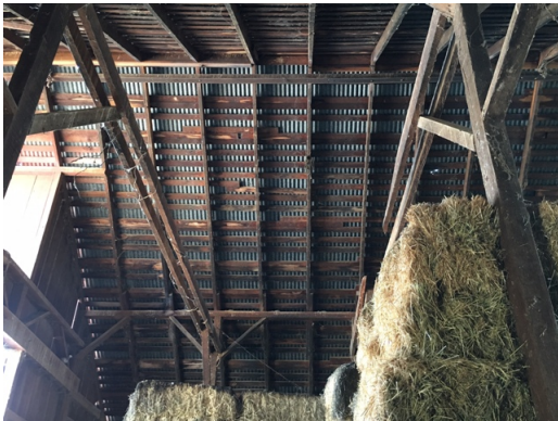
Dillard Ranch - Barn2 - Roof Decking
