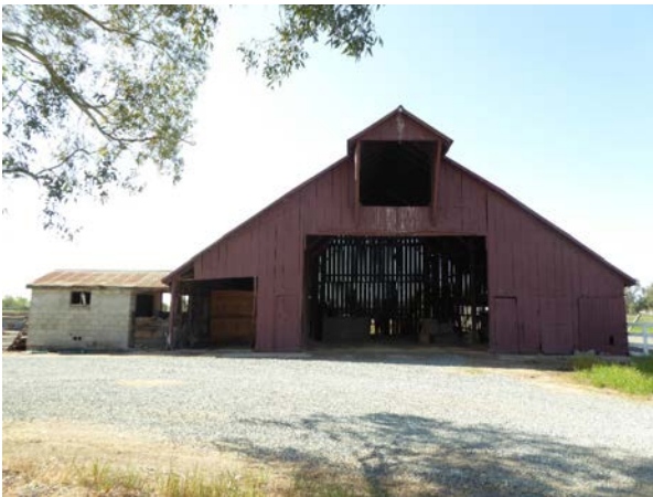
Figure 11: Looking south toward hay barn 1.
