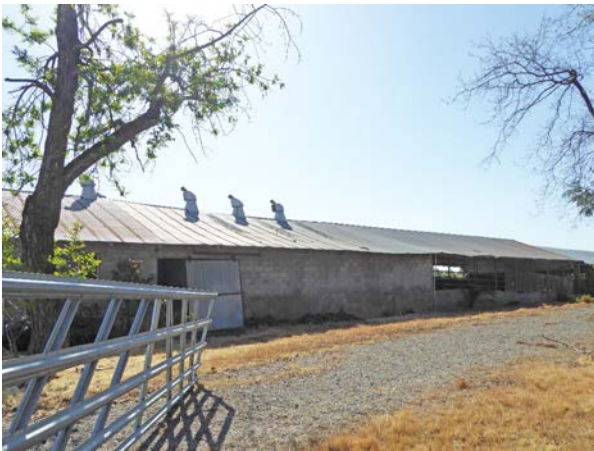
Figure 31: Concrete block section of the east façade, looking southeast.
