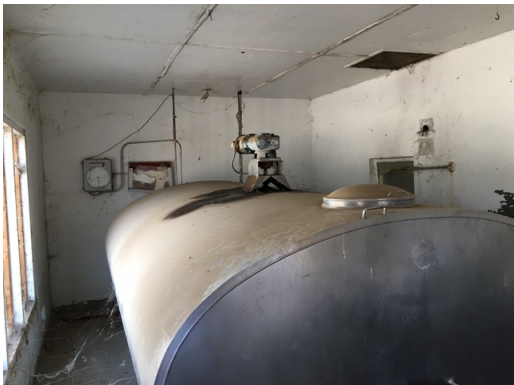
Dillard Ranch - Outbuilding Shed - Interior Room
