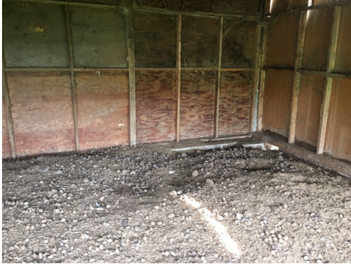
Dillard Ranch - Shed1 - Floor
