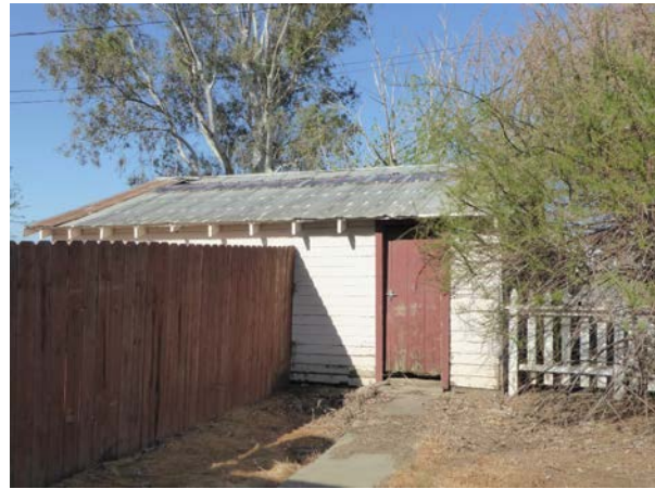
Figure 9: East façade, looking west.
