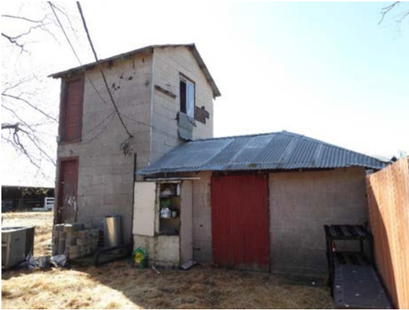
Figure 21: View of the tankhouse building, looking northwest.
