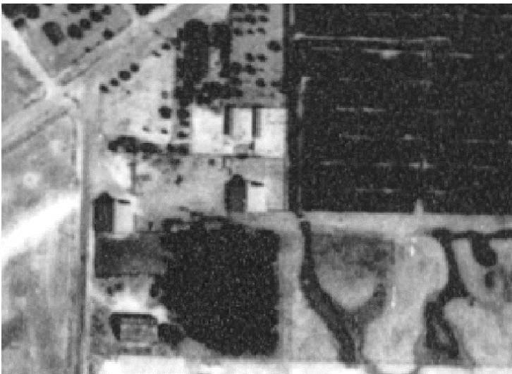
Figure 49: Detail view of buildings present at Dillard Ranch as of 1937.
