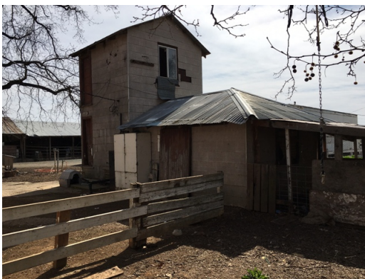
Dillard Ranch - Well Pump - Northwest
