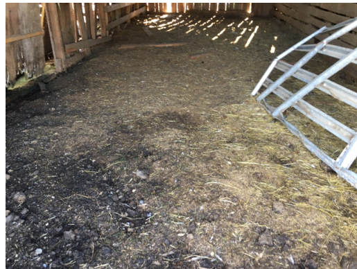
Dillard Ranch - Barn2 - Dirt Floor
