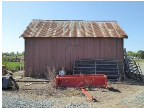
Figure 20: Looking south at north façade of granary with door cut into board-and-batten siding.
