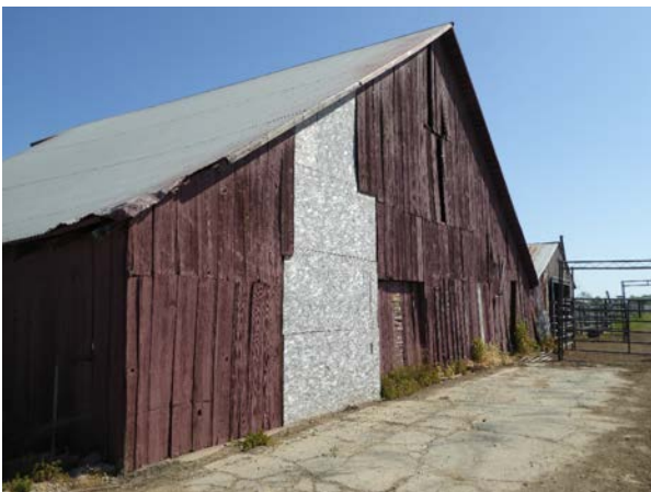
Figure 17: Rear façade of hay barn 2, looking east.
