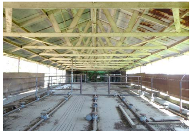
Figure 34: Dairy barn, to the south of the milker's pit, looking north.
