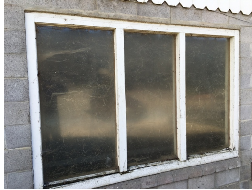
Dillard Ranch - Outbuilding Shed - Wood Frame Windows
