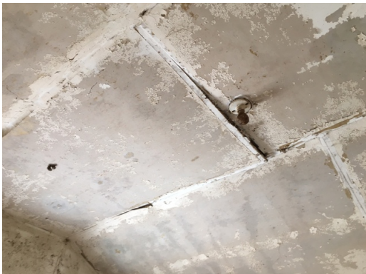
Dillard Ranch - Well Pump - Second Floor Ceiling
