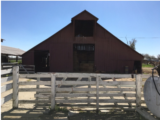
Dillard Ranch - Barn2 - North Elevation
