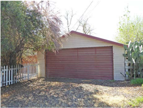
Figure 8: Front of garage, looking south.
