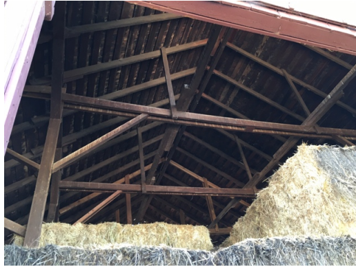
Dillard Ranch - Barn1 - Roof Decking
