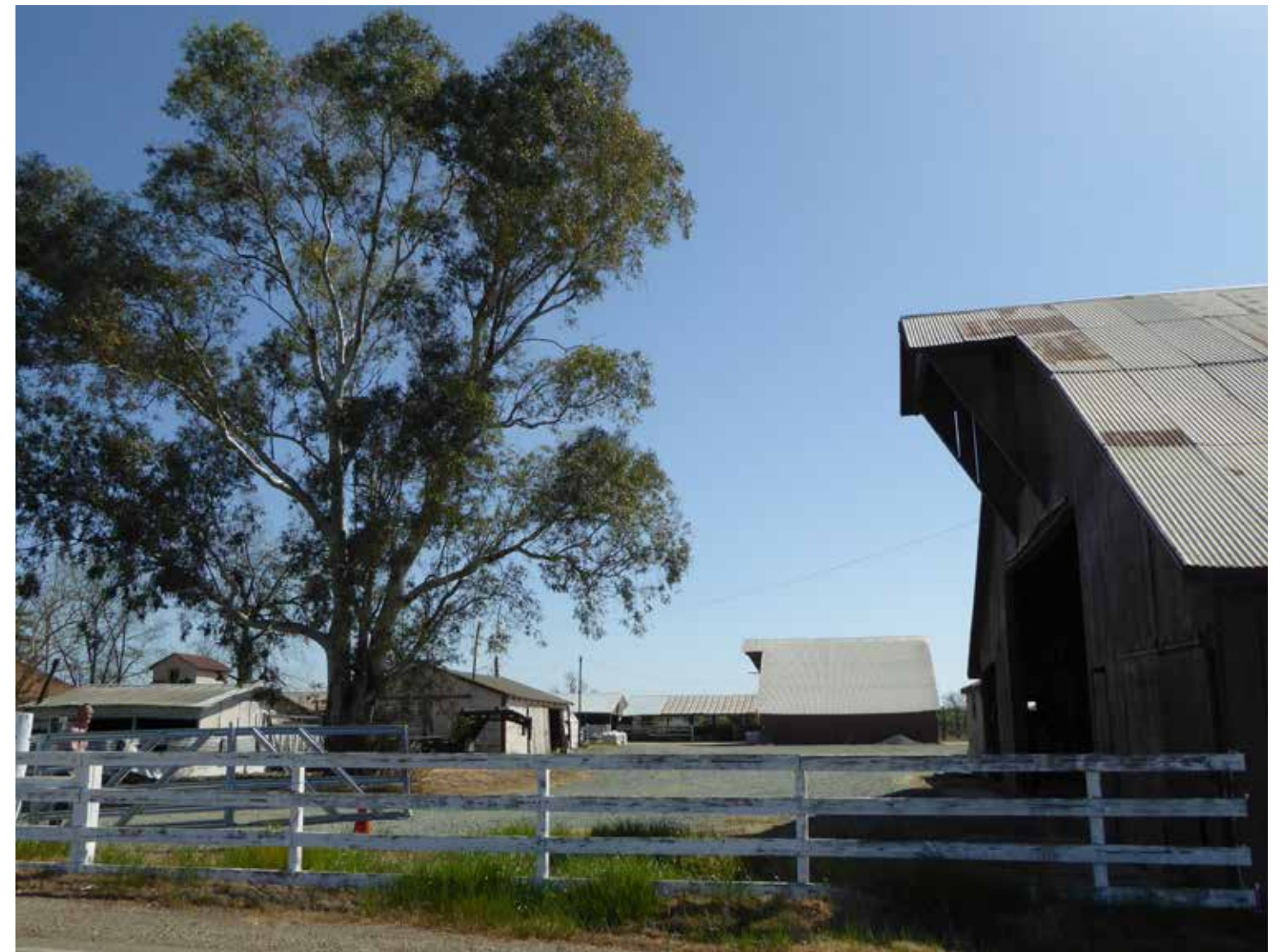
Figure 10: Hay Barn 2 and other agricultural buildings at the rear of the historic building cluster, view east.
