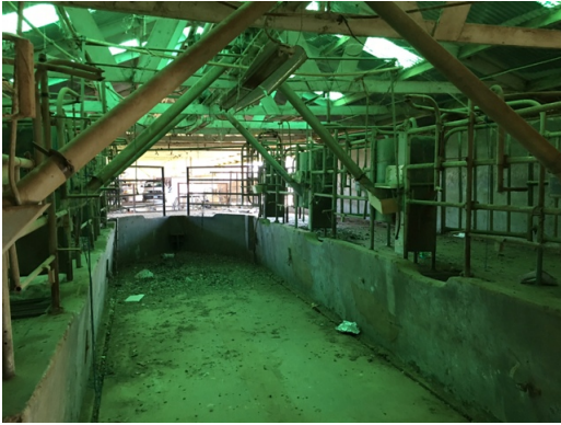
Dillard Ranch - Outbuilding Shed - Milk Stations
