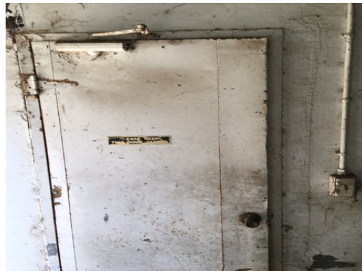
Dillard Ranch - Outbuilding Shed - Interior Door
