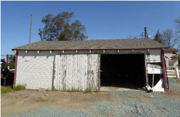
Figure 27: South façade of workshop, looking east.
