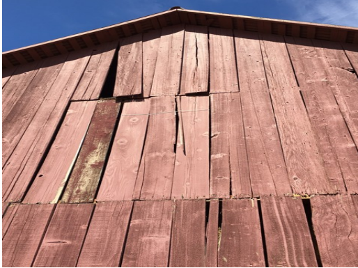
Dillard Ranch - Barn2 - Exterior Detail
