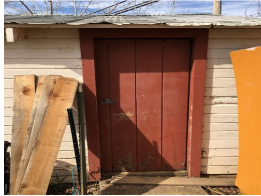
Dillard Ranch - Garage - Eastside Door
