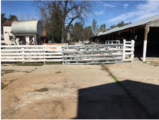
Dillard Ranch - Barn2 - Pavement
