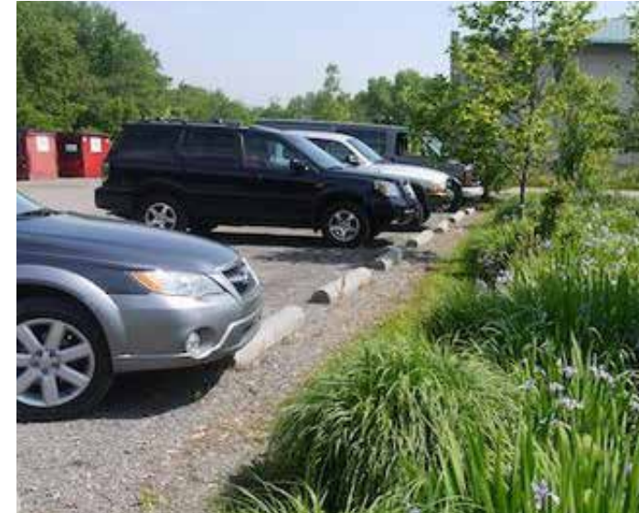
Figure 50: Parking area with timber wheel stops.
