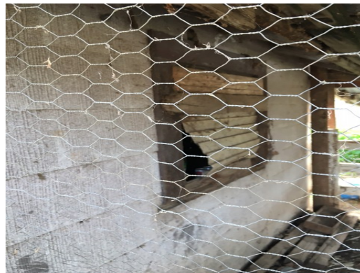
Dillard Ranch - Well Pump - Window
