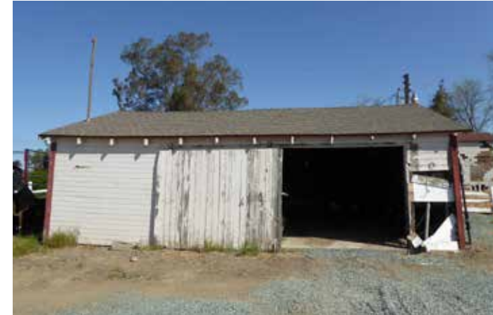
Figure 21: The Storage Shed to be replaced by a new public restroom.
