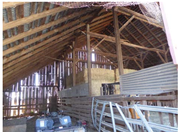
Figure 18: Interior truss system at hay barn 2.
