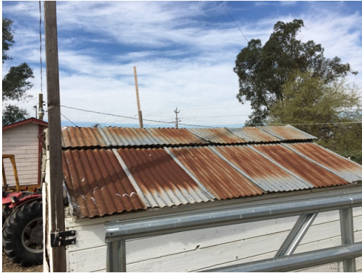
Dillard Ranch - Outbuilding1 - Roof
