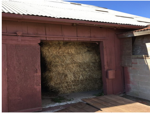
Dillard Ranch - Barn1 - Sliding Door
