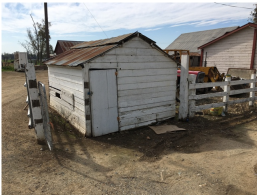
Dillard Ranch - Outbuilding1 - North Elevation
