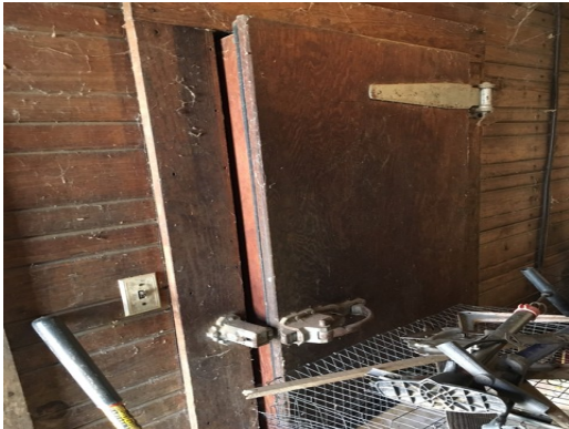
Dillard Ranch - Well Pump - Food Storage
