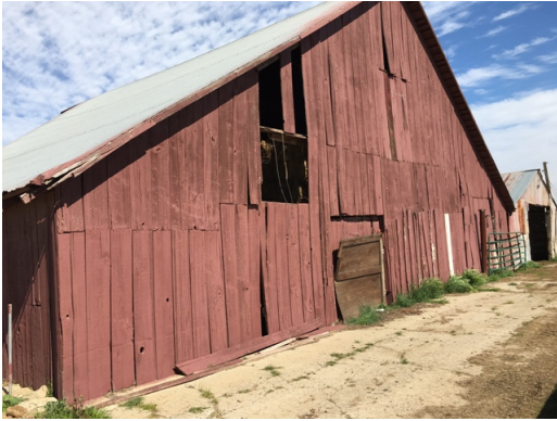
Dillard Ranch - Barn2 - South Elevation
