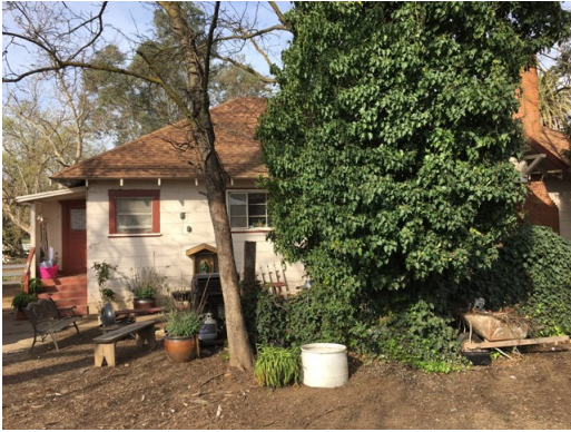
Dillard Ranch - House - East Landscaping
