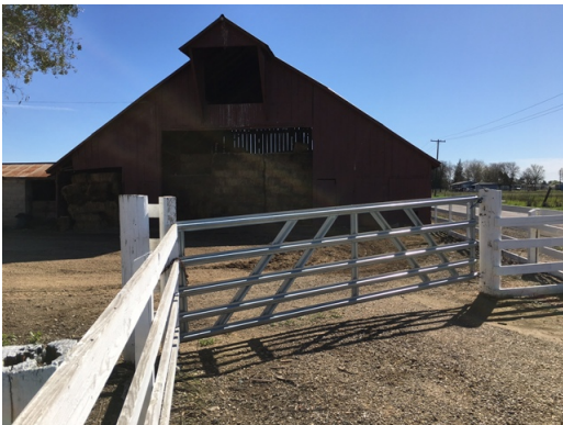
Dillard Ranch - Barn1 - Gate
