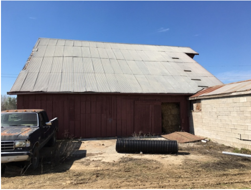
Dillard Ranch - Barn1 - Roof
