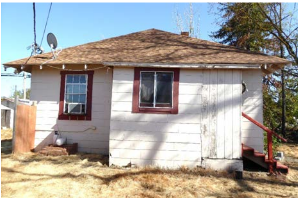
Figure 6: Rear façade of the ranch house, with shed porch addition.
