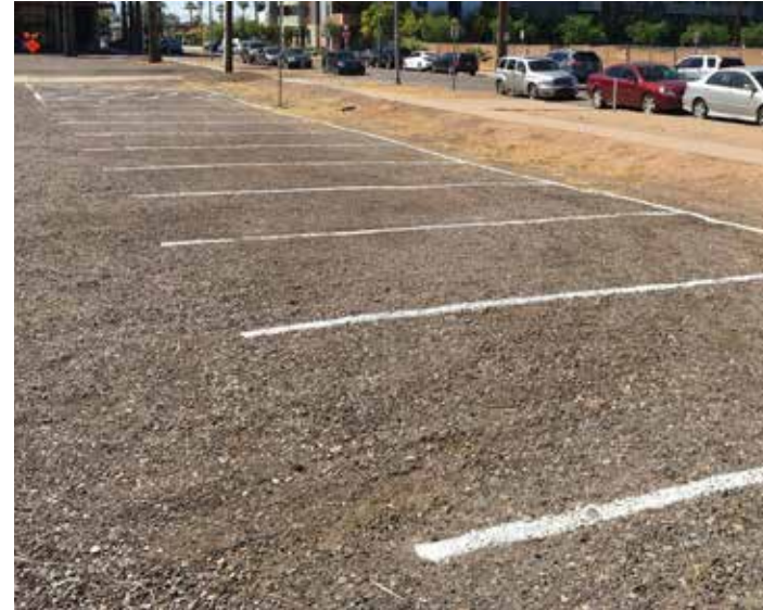
Figure 49: Compacted gravel parking area.
