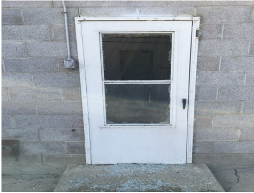
Dillard Ranch - Outbuilding Shed - Exterior Door
