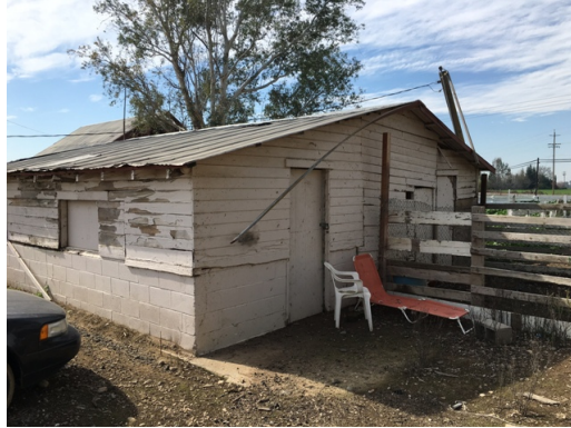
Dillard Ranch - Shed1 - North Exterior
