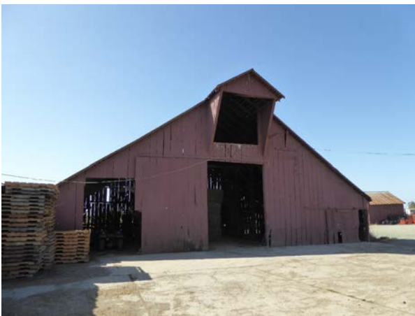
Figure 15: North façade of hay barn 2, looking south.
