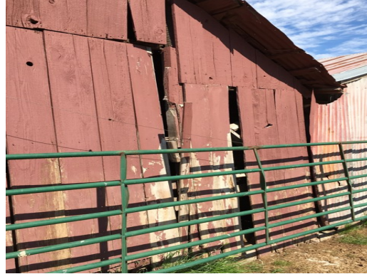
Dillard Ranch - Barn2 - Exterior Detail
