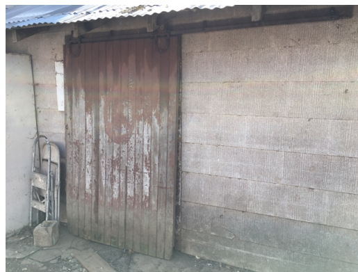
Dillard Ranch - Well Pump - Sliding Door
