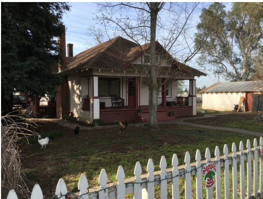
Dillard Ranch - House - North Elevation
