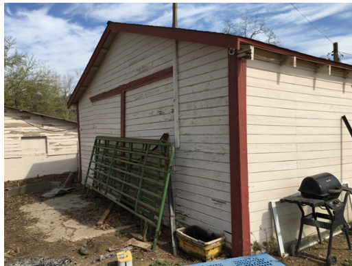
Dillard Ranch - Outbuilding2 - East Exterior
