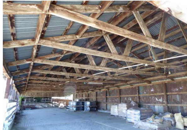
Figure 35: Southern end of the dairy barn, looking north.
