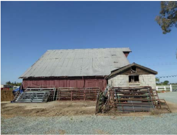
Figure 13: East façade of hay barn 1, looking west.
