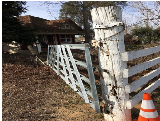
Dillard Ranch - House - Drive Gate
