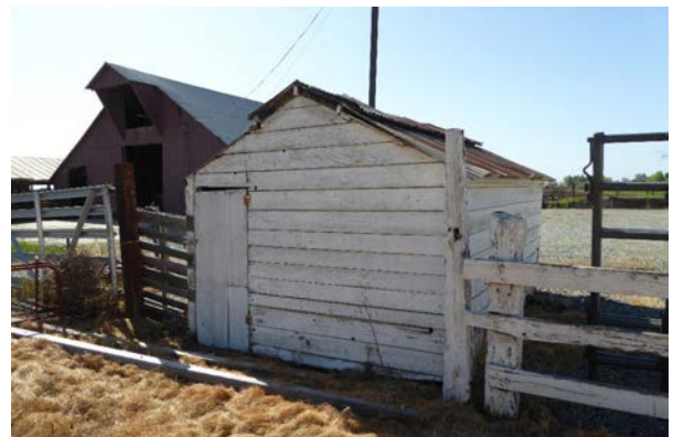
Figure 24: North façade of the small storage shed, looking southeast.
