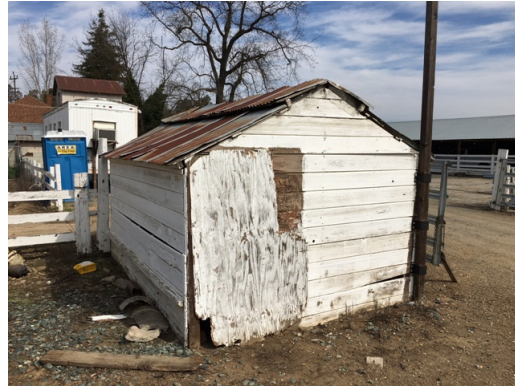
Dillard Ranch - Outbuilding1 - South Elevation
