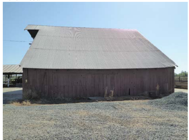
Figure 16: Looking east at west façade of hay barn 2.
