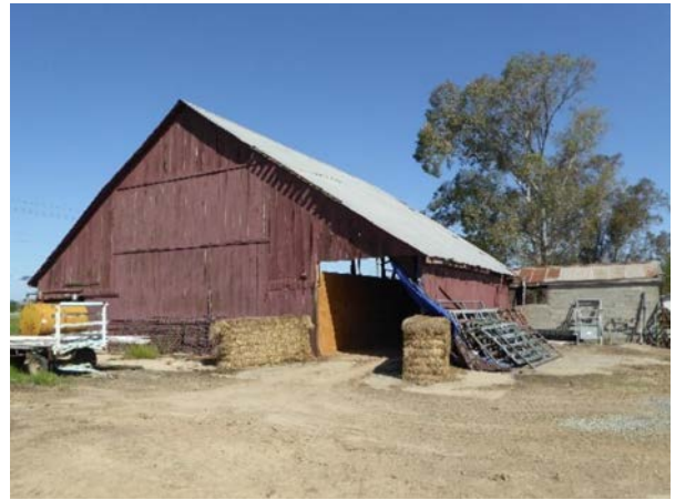
Figure 14: Rear façade of hay barn 1, looking northwest.
