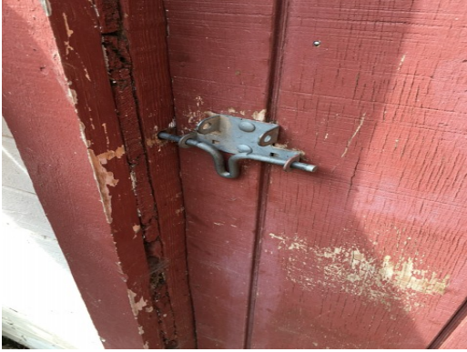
Dillard Ranch - Garage - Door Hardware
