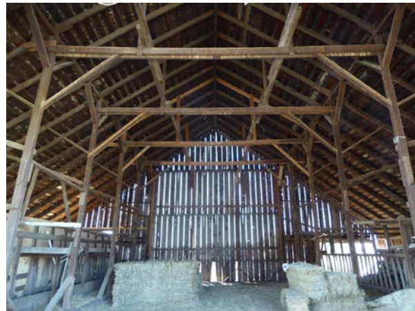
Figure 12: Wood truss structural system, looking south.
