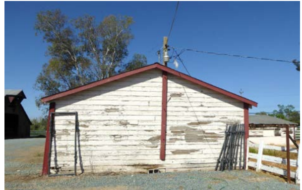
Figure 28: East façade of workshop, looking west.
