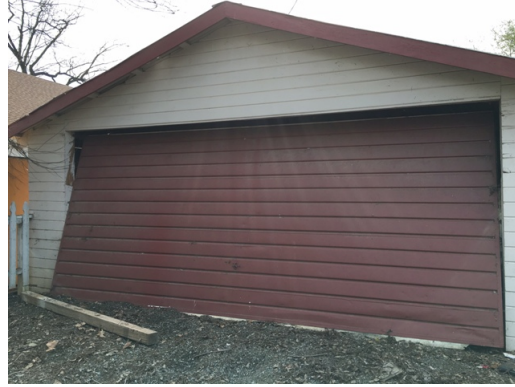
Dillard Ranch - Garage - Garage Door
