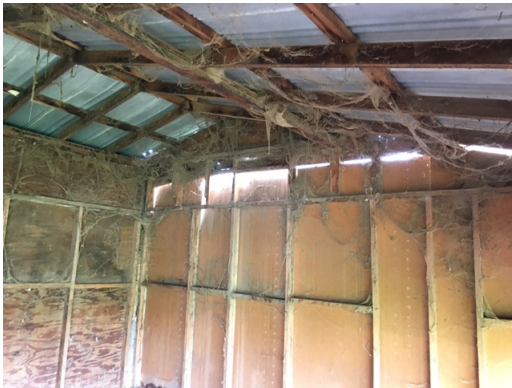
Dillard Ranch - Shed1 - Interior
