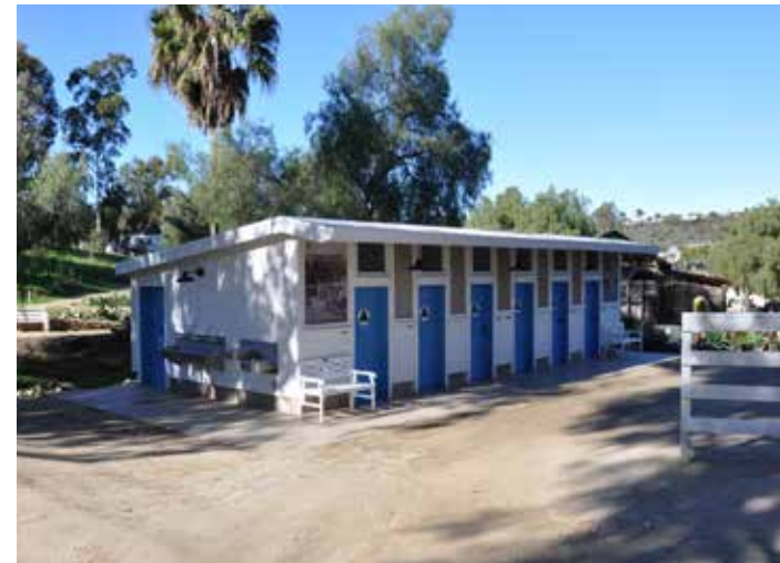
Figure 26: New restroom at Leo Carillo Ranch, modeled after a chicken coop that previously stood in the same location.
