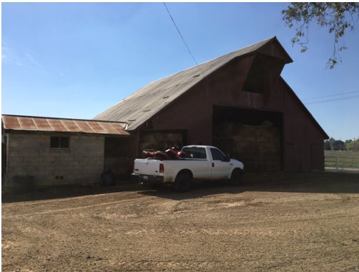
Dillard Ranch - Barn1 - Elevation
