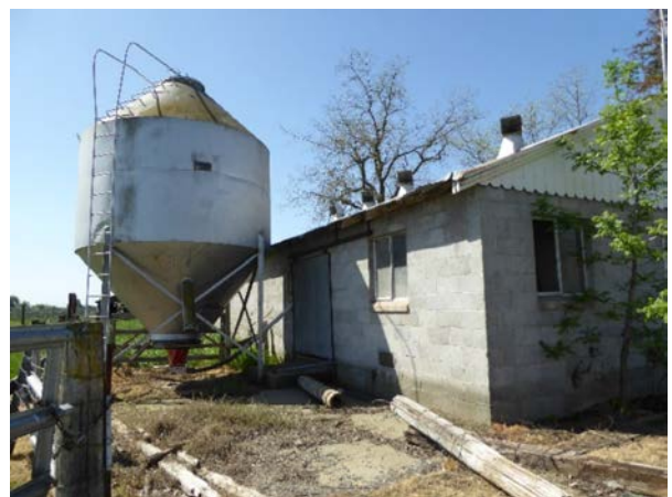
Figure 30: Feed hopper next to east façade, looking south.
