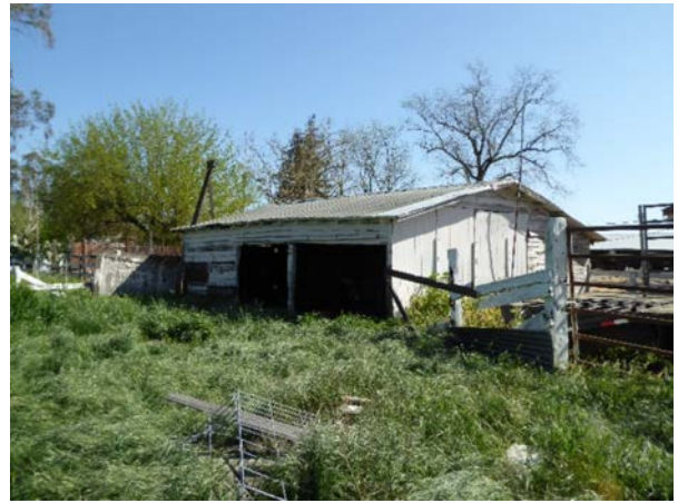
Figure 26: West (left) and south (right) façades, looking north.
