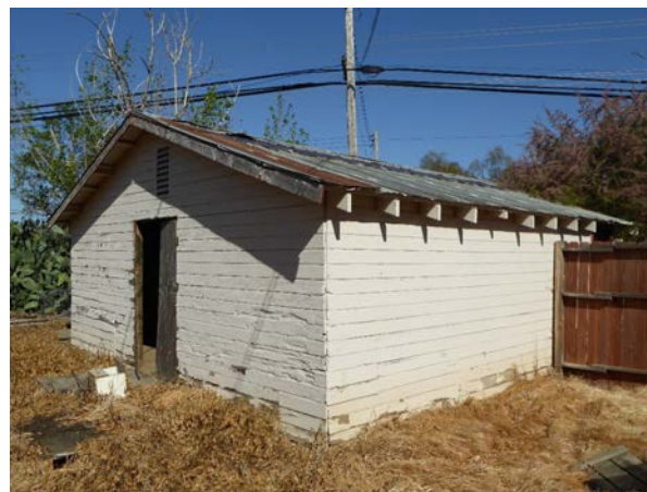
Figure 10: Rear of garage, looking northwest.
