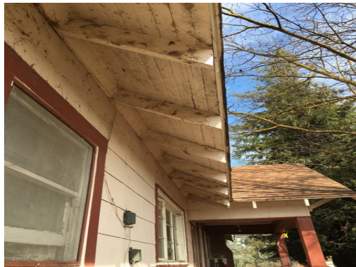
Dillard Ranch - House - Soffit
