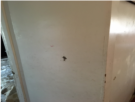
Dillard Ranch - House - Interior Wall
