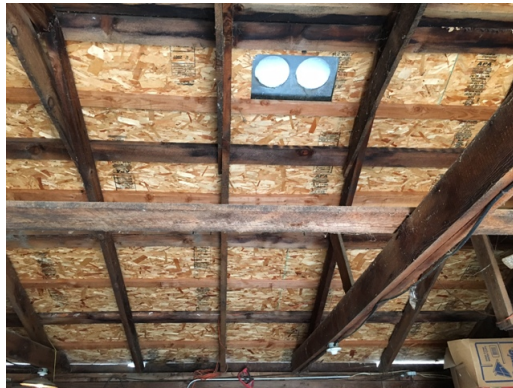
Dillard Ranch - Outbuilding2 - Roof Decking
