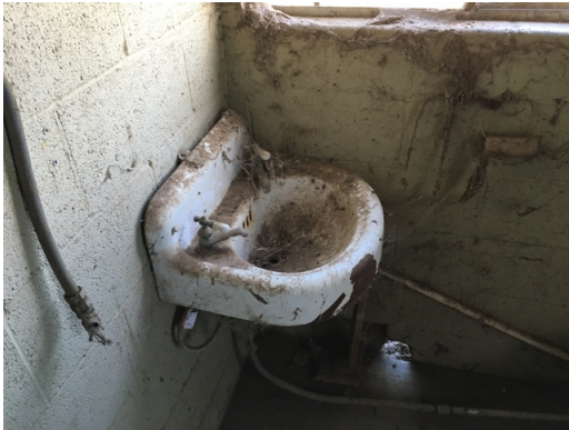
Dillard Ranch - Outbuilding Shed - Sink
