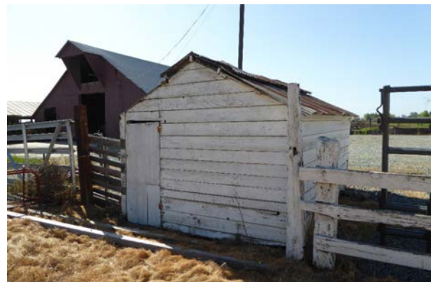
Figure 24: North façade of the small storage shed, looking southeast.
