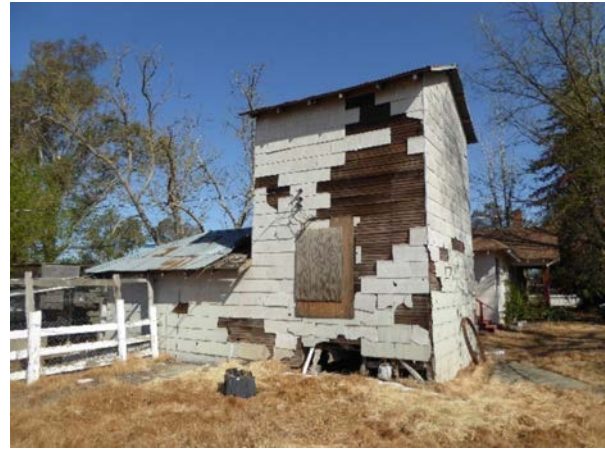
Figure 22: South façade of tankhouse, looking north.
