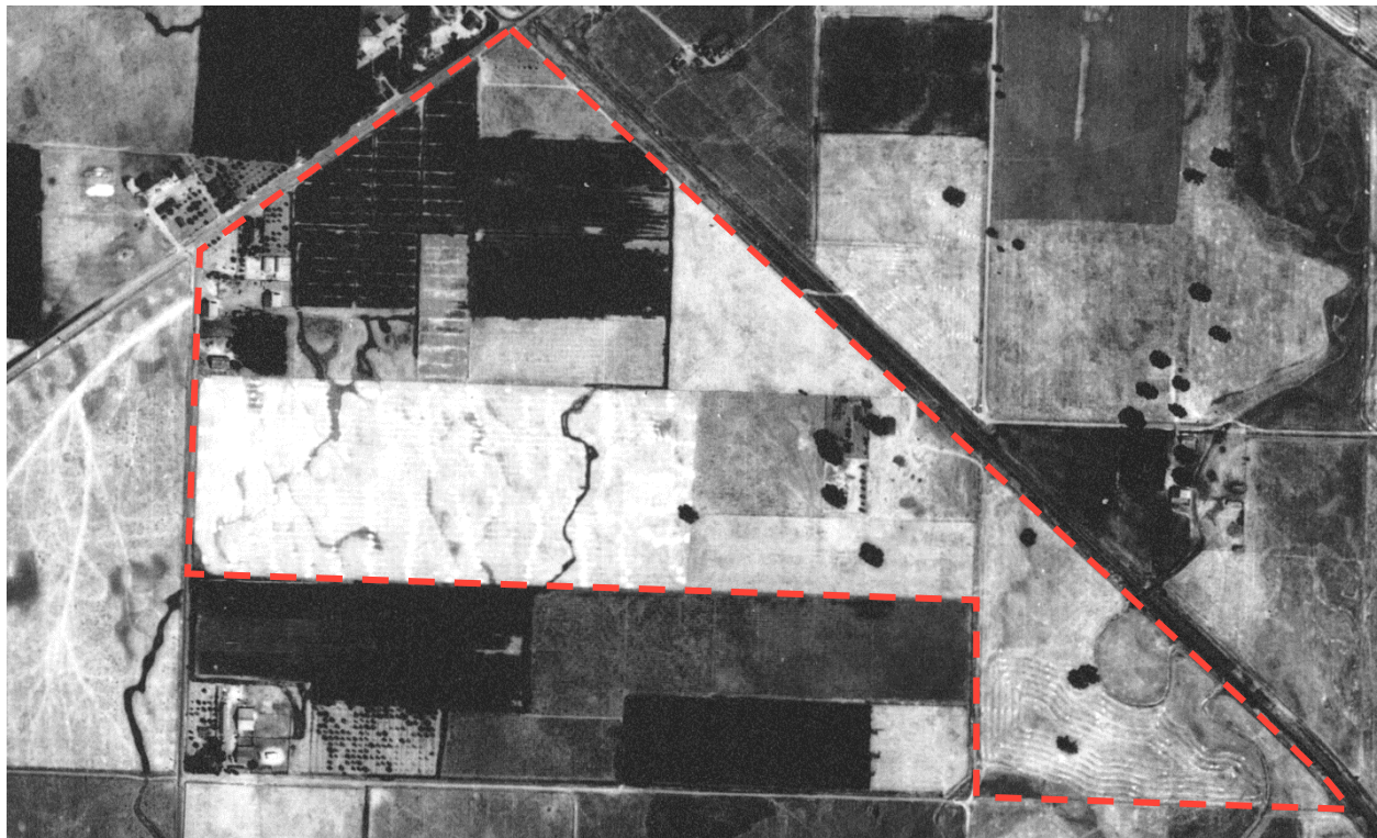
Figure 48: Aerial view of Dillard Ranch (approximate property boundaries outlined in red, 1937. Cluster of buildings within the ranch appear at upper left. Source: UC Santa Barbara Frame Finder, ABC-1937-45-79. Edited by Page & Turnbull.
