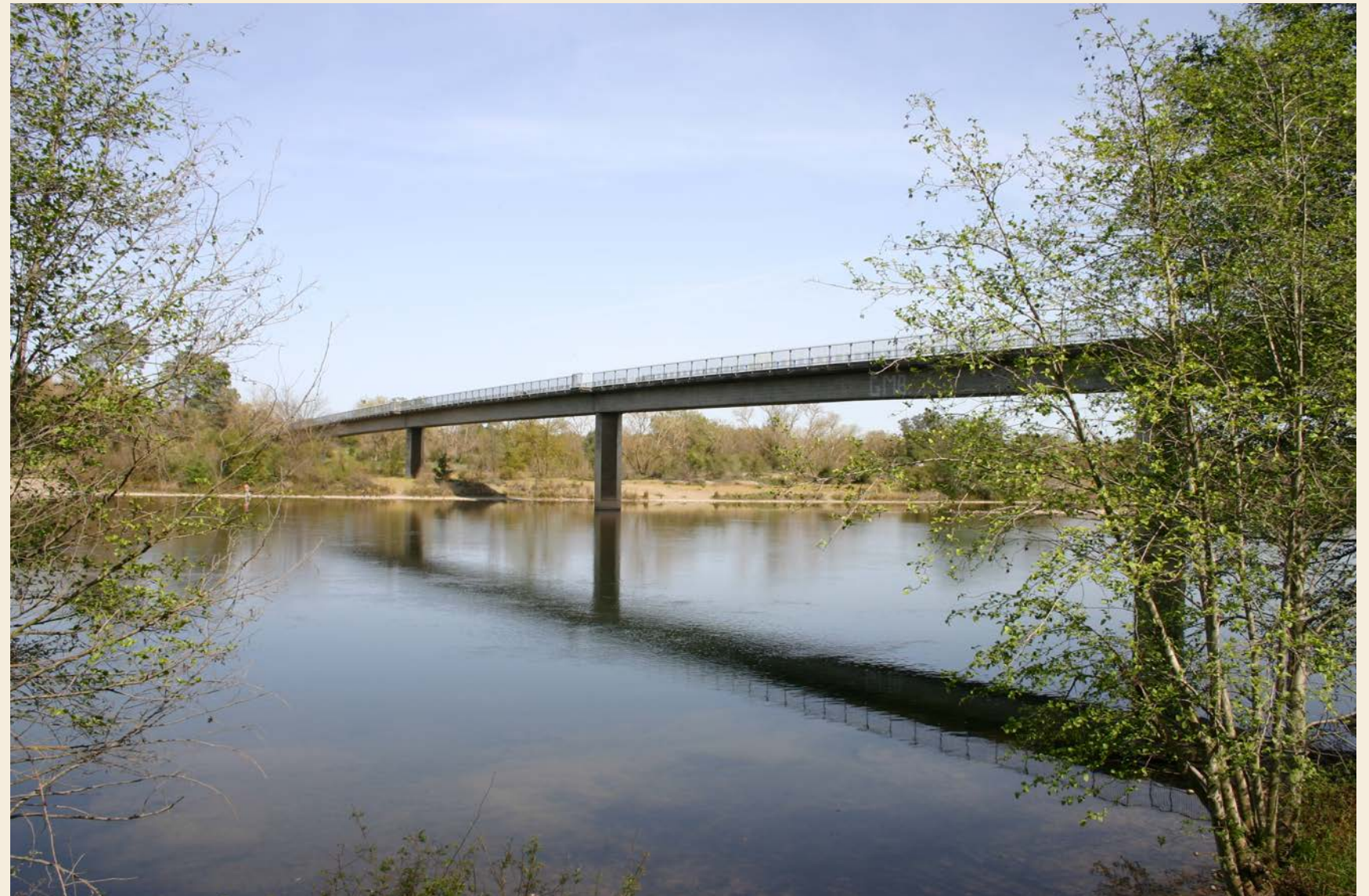
The Harold Richey Memorial Bicycle Bridge in the Arden Bar and River Bend Park Areas. Photo Credit: Regional Parks
