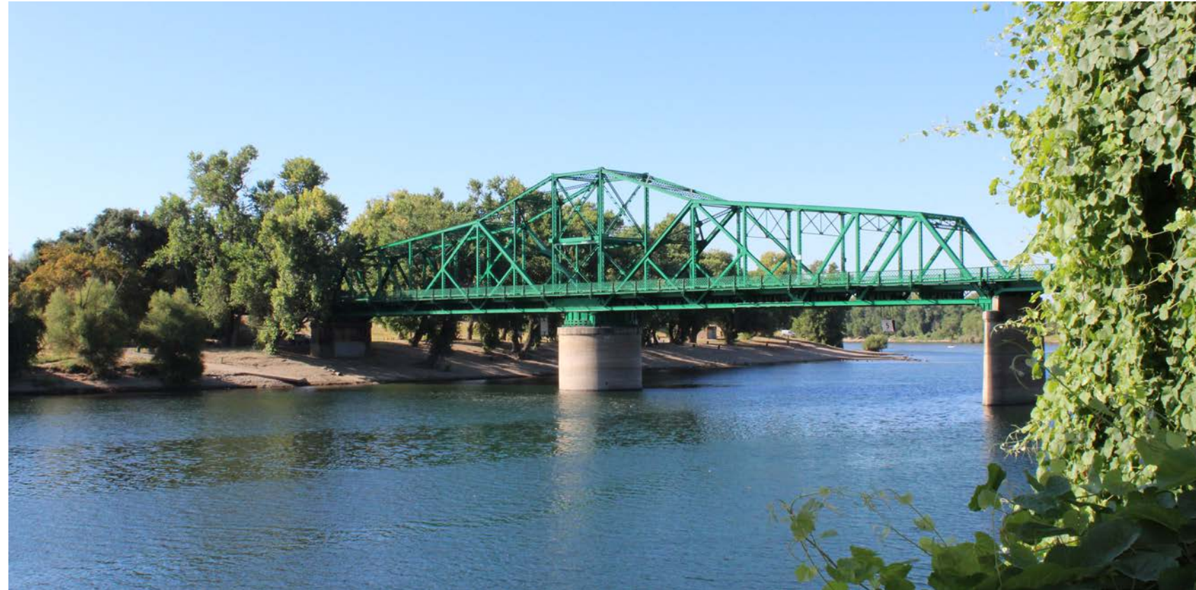
The Jibboom Street Bridge in the Discovery Park Area. Photo Credit: MIG
