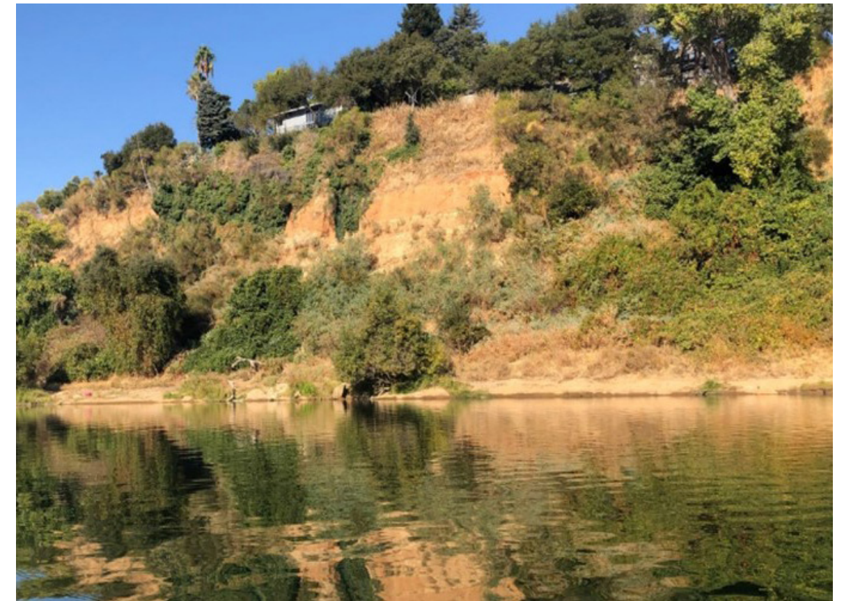
FIGURE 5-23 STEEP BLUFFS ALONG RIGHT BANK (~RM 19.4)
