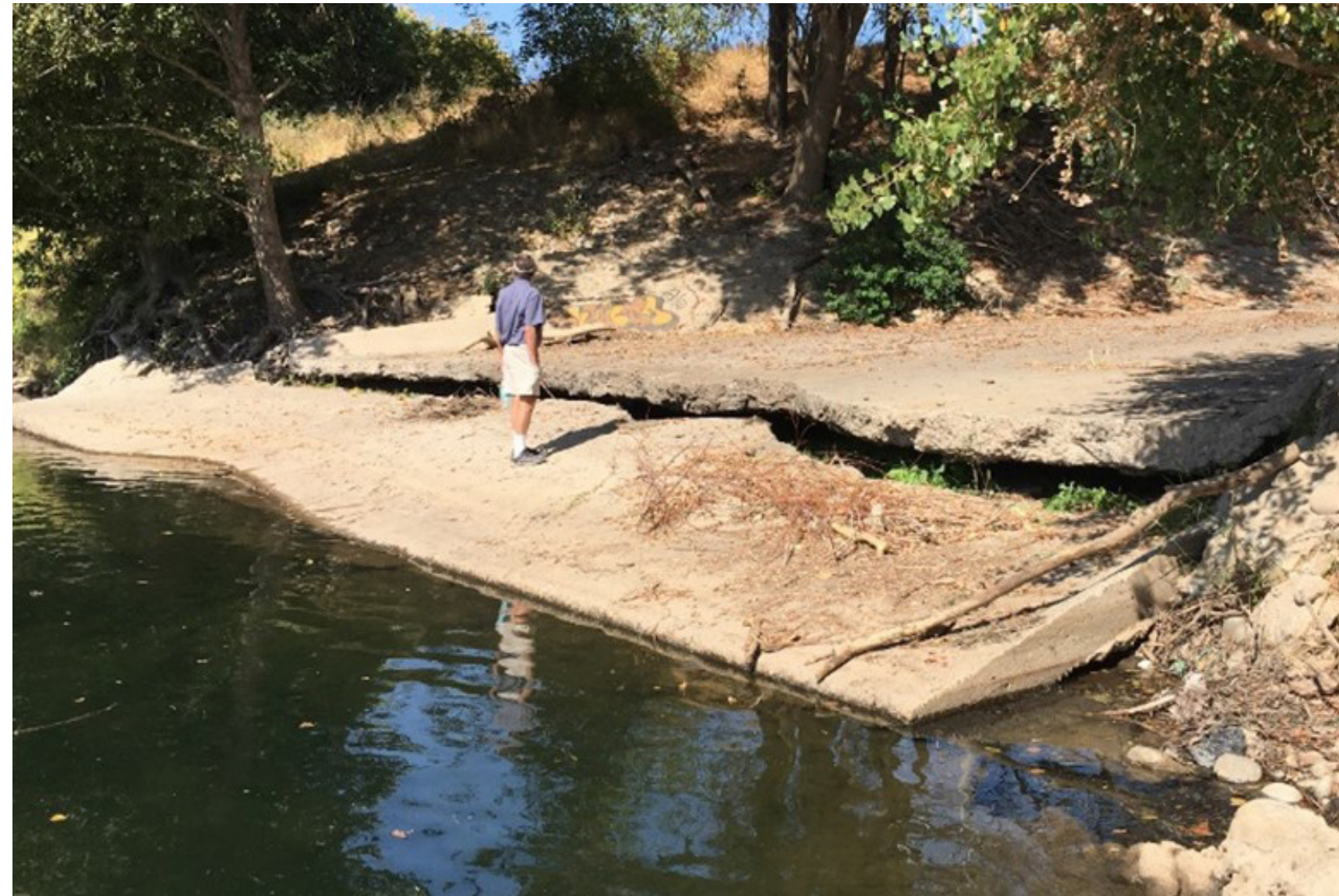
FIGURE 5-12 LARGE URBAN STORMWATER OUTFALL WITH BROKEN APRON (~RM 5.3)
