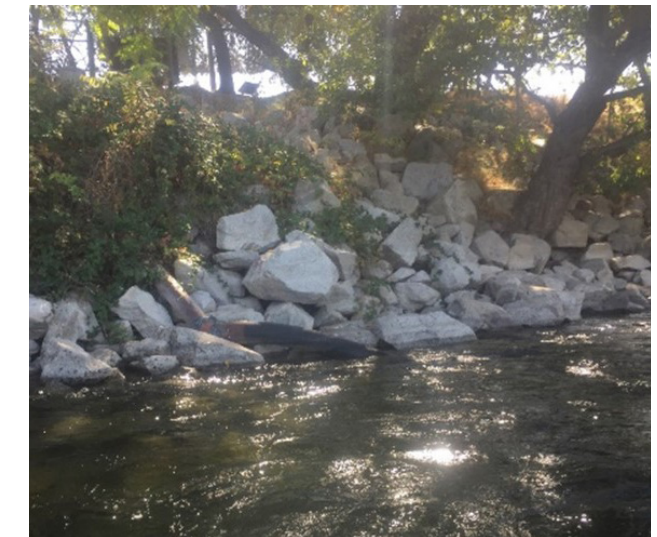
FIGURE 5-21 ROCK RIP-RAP PLACED AT CORDOVA CREEK OUTFALL (~RM 14.5)
