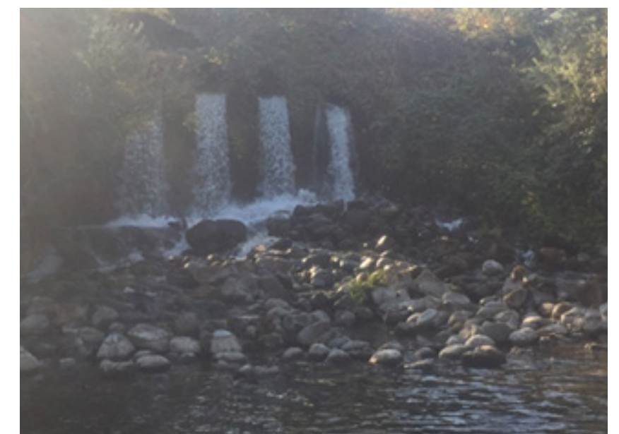
FIGURE 5-24 BUFFALO CREEK OUTFALL (~RM 19.5)
