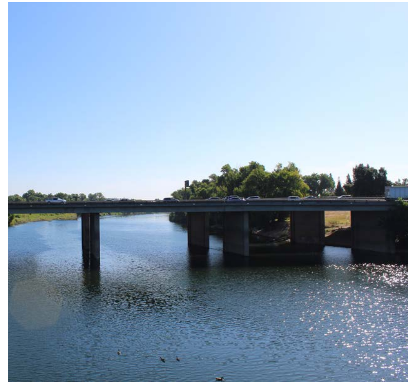
The I-5 American River Bridge in the Discovery Park Area. Photo Credit: MIG
