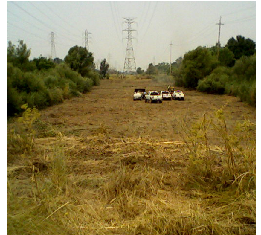
Vegetation clearing activities under WAPA powerlines in the Cal Expo Area. Photo Credit: Regional Parks
