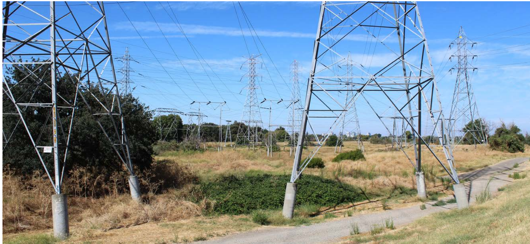
Electrical power transmission towers in the Cal Expo Area. Photo Credit: MIG
