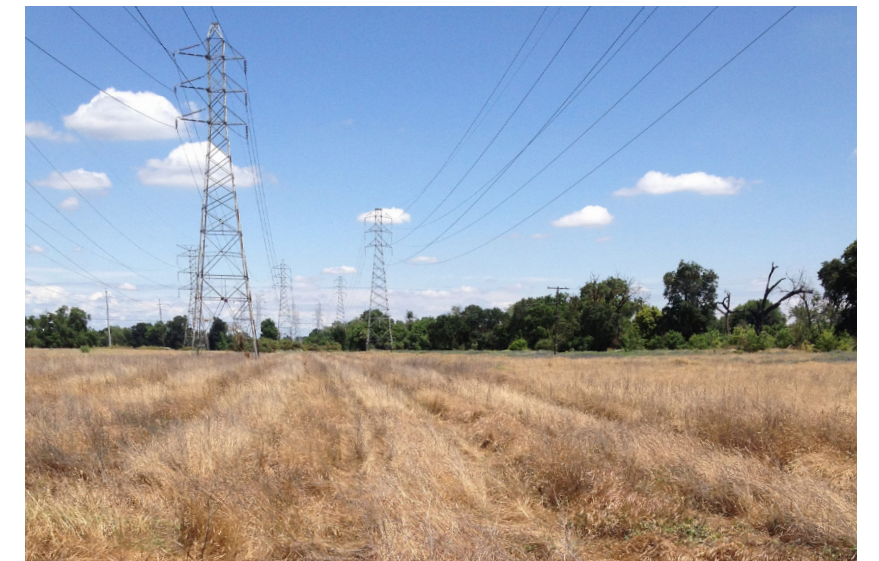
Powerline easement in the Woodlake Area. Photo Credit: Regional Parks
