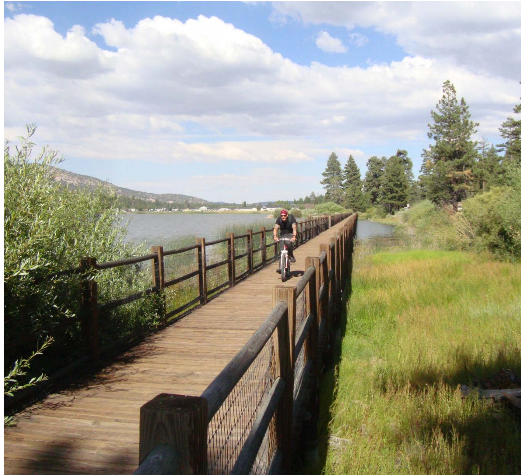
The Stanfield Marsh Boardwalk, an example of environmentally-friendly raised platform trail design. Photo Credit: MIG
