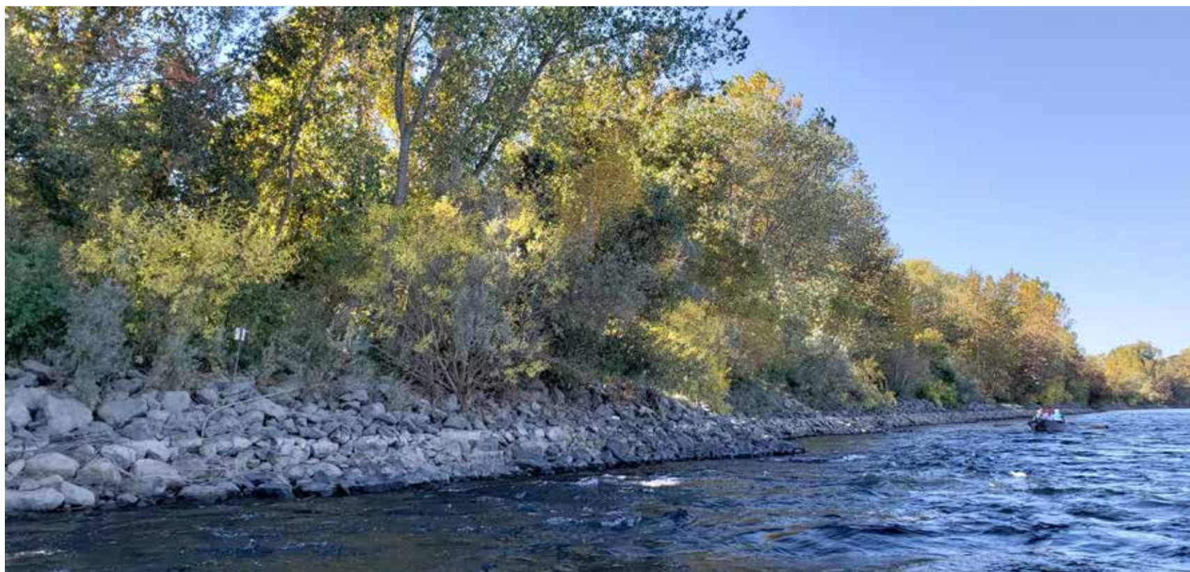
Revetment and riparian plantings along riverbank. Photo Credit: KC Sorgen
