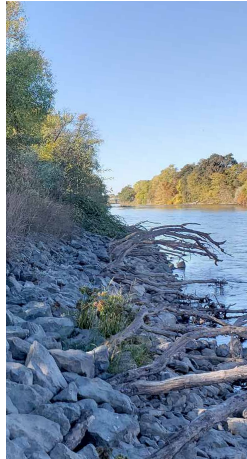
Revetment and riparian plantings along riverbank. Photo Credit: KC Sorgen
