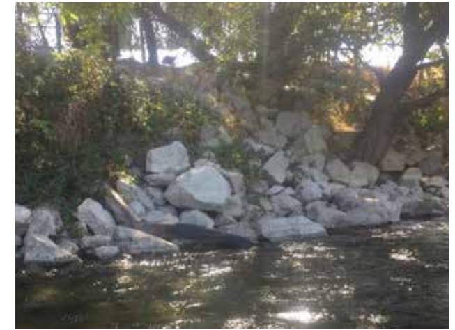
FIGURE 5-25 ROCK RIP-RAP PLACED AT CORDOVA CREEK OUTFALL (~RM 14.5)
