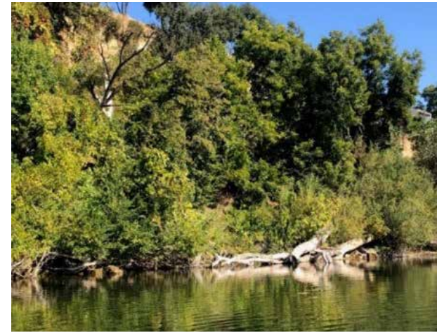
FIGURE 5-24 ACTIVELY ERODING BANK ALONG CLAY SHELF (~RM 17.8)
