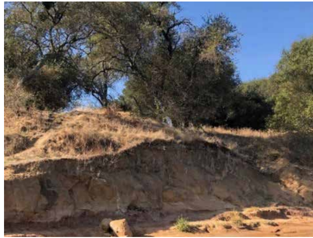
FIGURE 5-23 EROSION ALONG CLAY SHELF (~RM 16.7)
