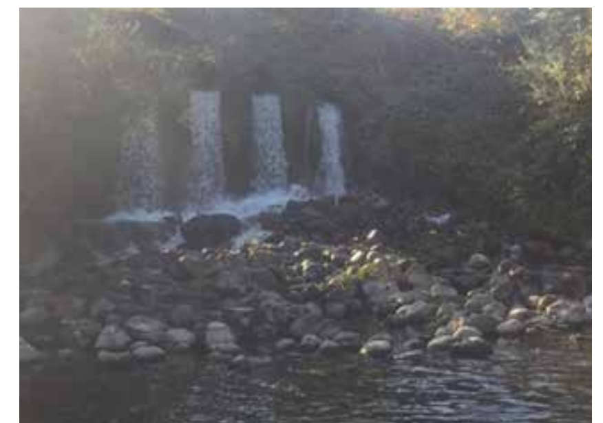
FIGURE 5-29 BUFFALO CREEK OUTFALL (~RM 19.5)
