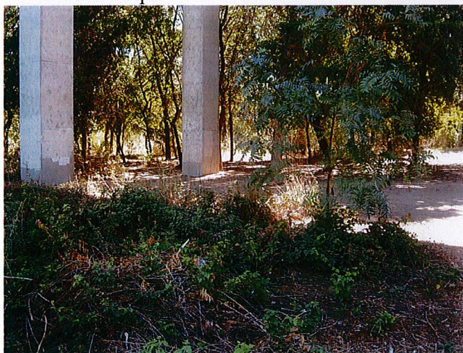
4E. Native plants next to cleared area under bridge
